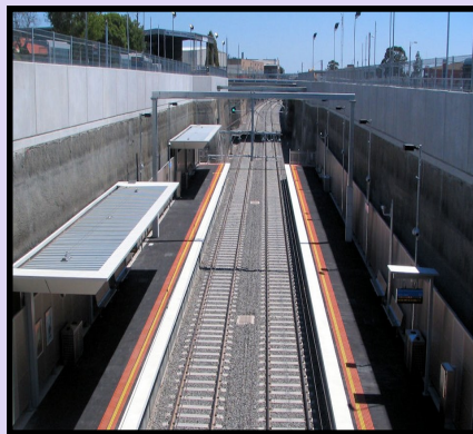
Photo of Lowered Rail Line at Mitcham Station, opened January 2014
